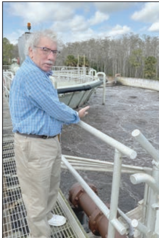
Glenn standing atop the wastewater plant biological aeration basin.
